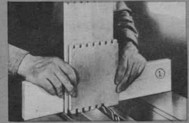
Cut box joints with a dado head.
